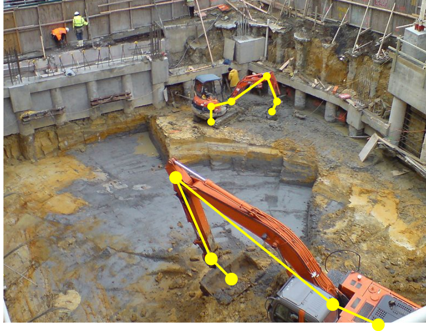
Figure 3-1: In this motivating construction site example, the two excavators must be tracked and avoided by an autonomous system. Yellow lines shows a notional kinematic chain provided as input to our tracking system.
